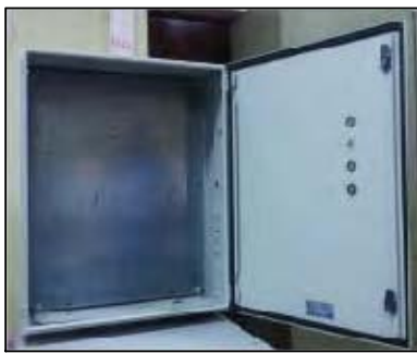
CONTROL PANEL WITH MOUNTING AND FIXING HOLES
